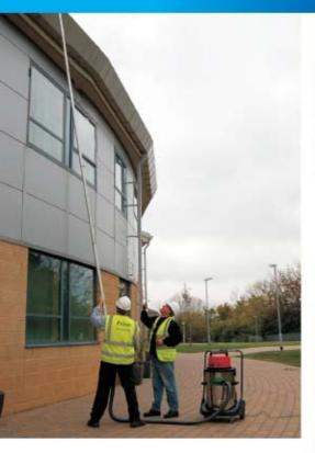
These are then connected to a powerful vac system which allows debris in the gutters to be sucked out.
